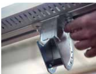
Step 1. Install the bracket
